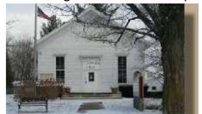
Hadley Township Town Hall
